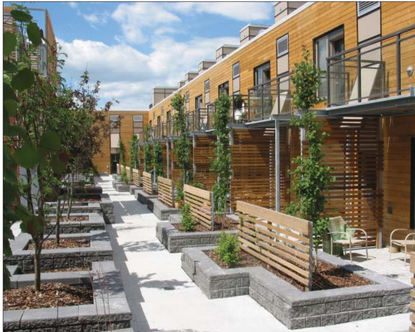
The two-story residential units at the Vento in Calgary, Alberta, open onto a shared courtyard, providing residents with access to the outdoors. The balconies also provide shading for the lower levels of the units.
